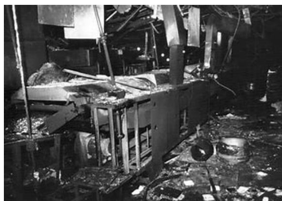
The area where the hydraulic hose was replaced
