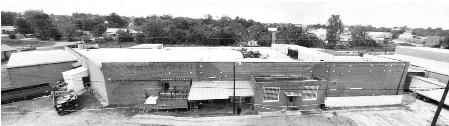
An aerial view of the Imperial Food Product Plant in Hamlet, North Carolina
