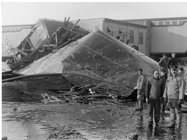
A section of the tank after explosion
